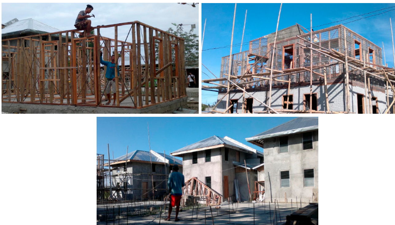
Figure 2. Construction of ten two-story duplex houses, Iloilo City, March 2015 [11].
