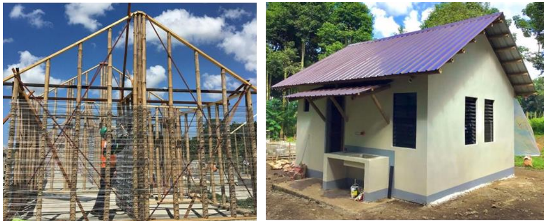
Figure 2. Single-family house using CBF technology in the Philippines (source: Base Bahay).
