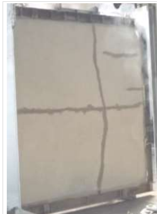
Figure 8. Specimen M2 condition after testing on the fire-exposed side. The black line is grouted to cover hair cracks before the burning test
