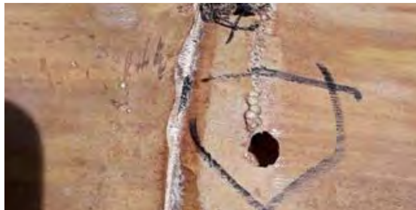
Visible exit hole (between 1 and 6 mm diameter) due to longhorn beetle damage.
