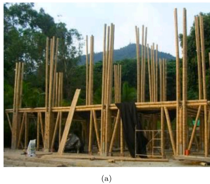
Fig. 18. Typical round bamboo member: (a) beam and column in framing system; (b) stud or brace in CBFT wall. Adapted from Archila-Santos et al. [283] and Bundi et al. [281], respectively.
