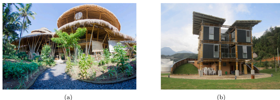
Fig. 32. (a) The Heart of School building at Green School Bali, Indonesia. After IBUKU [468]. (b) Energy-efficient bamboo house in Baoxi, China. After Laverde [413].
