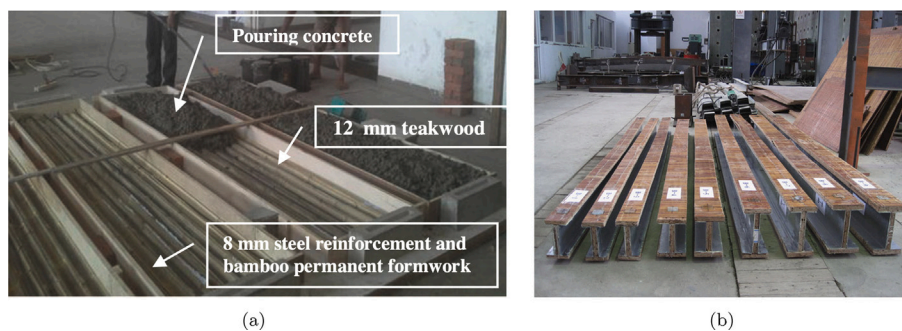
Fig. 38. (a) Bamboo permanent formwork during the casting of concrete. After Akmaluddin et al. [505]. (b) Bamboo-steel composite beam specimens. After Li et al. [510].
