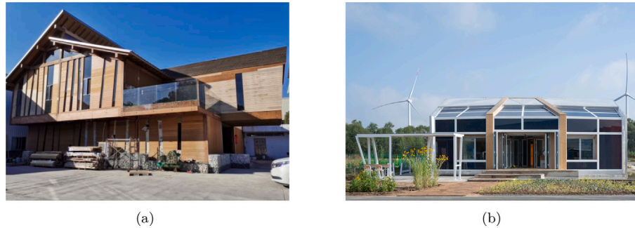
Fig. 34. (a) Building of Sentai bamboo research Center, GanZhou, China. After Su et al. [472]. (b) Y-Project building presented at the Solar Decathlon China (SDC) 2022 in Zhangjiakou, China. After Han [475].
