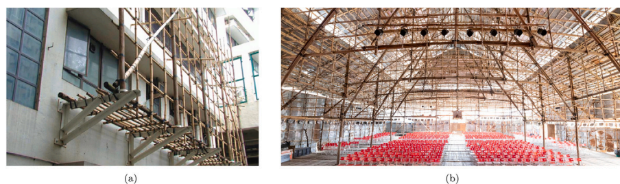
Fig. 27. (a) Steel bracket support for bamboo scaffolding. After Ramanathan [452]. (b) A bamboo theatre building in Hong Kong [453].
