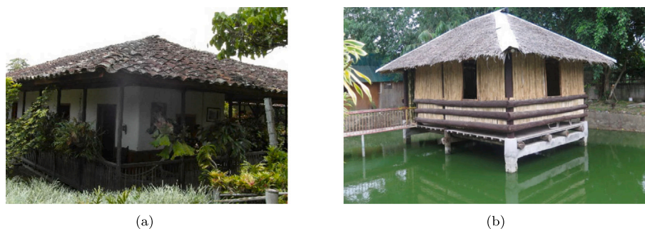
Fig. 31. Examples of (a) traditional bahareque house in Armenia, Colombia. After Kaminski et al. [466]. (b) Stilted bamboo house in the Philippines. After De Araujo et al. [448].
