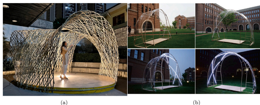
Fig. 28. (a) A bending-active bamboo shell structure (BABSS) serving as a temporary urban pavilion. After Jiang et al. [457]. (b) full-scale temporary sheltered pathway module prototype in the spatial configuration in the campus garden during daytime (top) and at night with LED lighting (bottom). After Wang et al. [458].
