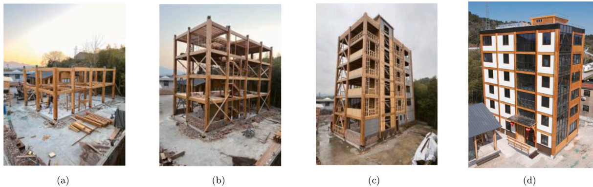
Fig. 35. The assembly construction process of the seven-story bamboo structure. (a) First and second floor construction unit; (b) third and fourth floor construction unit; (c) completed seven-story structural frame; and (d) completed building. Adapted from Wu et al. [486].
